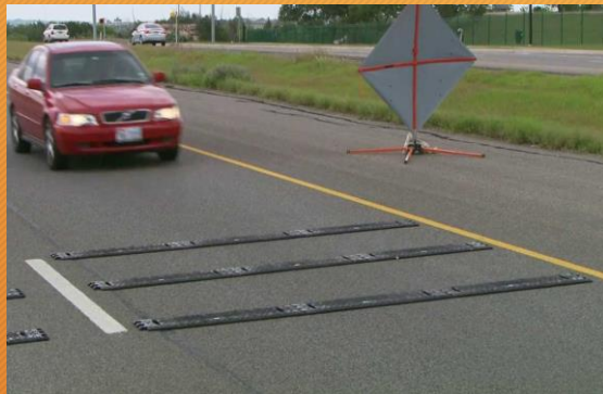
Temporary Rumble Strips
